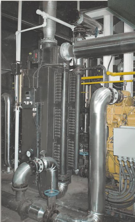
HOSPITAL, Ontario (2) Model HRSR-336B28CSS Recovering Btu from (2) Cummins Wartsila CW180, natural gas engines. Reducing each 968°F @ 3,666 SCFM to 339°F. Raising 175 GPM hot water from 195°F to 229°F.
