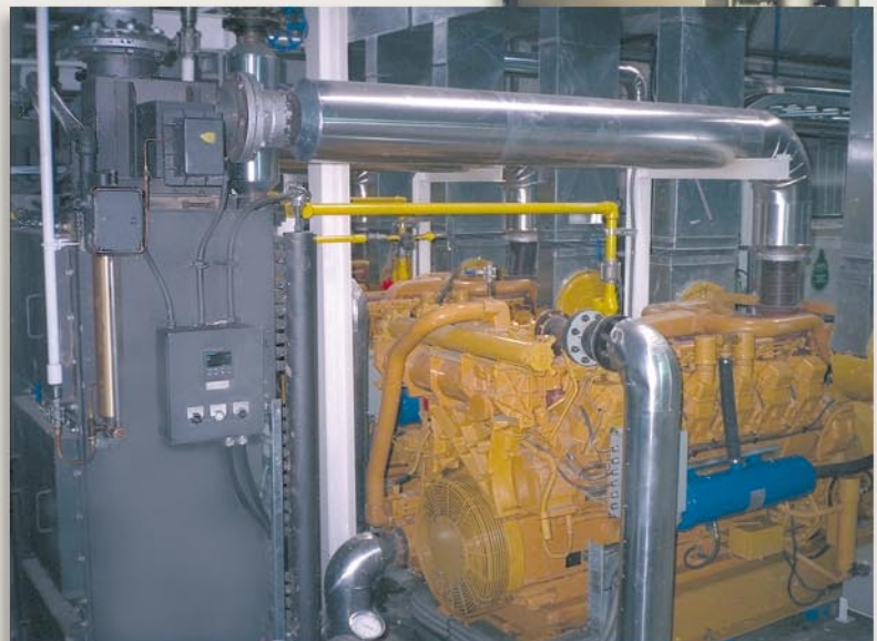
GOLD & SILVER MINE, Eskay Creek, British Columbia. (3) Model HRSR-316A26CSP Recovering Btu from (3) Caterpillar 3512, 900kW diesel engines. Reducing each 870°F @ 2,100 SCFM to 417°F. Raising 265 GPM 50% ethylene glycol from 187°F to 197°F.
