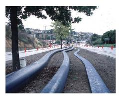
Features a unique "through-the-weave" one piece construction comprising a circular woven high tenacity polyester reinforcement totally encapsulated in a tough elastomeric polyurethane cover and lining. Manufactured in compliance with BS EN ISO 9001:2000 quality management systems. Raw materials, components, and finished products are rigorously tested and inspected to ensure excellent product reliability.
