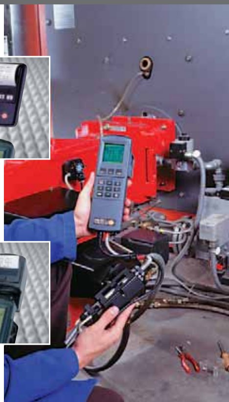
Burner tuning with testo 300 XL-I and mini gas preparation unit connected
