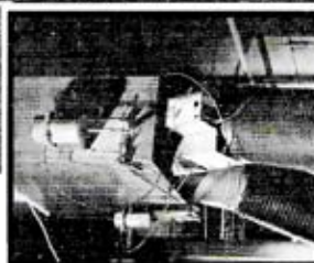
Southwestern Life Insurance, Dallas. Inset photos show Enviro-Master ® variable volume equipment used for retrofitting original medium pressure double duct system.
