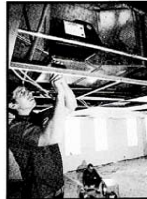
Park Tower South, Houston. Owner, Tenneco Realty, Inc. Major tenant, Exxon Chemical, U.S.A. Original constant volume reheat system retrofitted to variable volume. Total annual energy usage was reduced 38%. Consequently, owner ordered similar retrofit of building's twin, Park Tower North.
