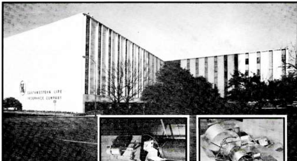
Southwestern Life Insurance, Dallas. Inset photos show Enviro-Master ® variable volume equipment used for retrofitting original medium pressure double duct system.
