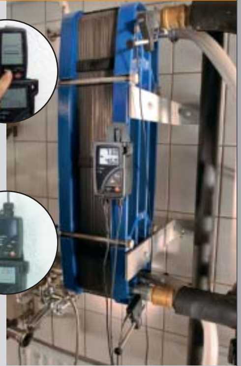
Checking technical systems (flow/return temperature) in production facilities
