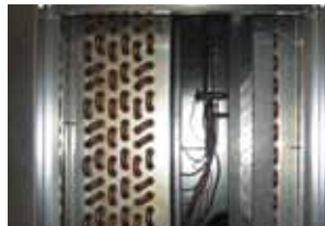
PDX & Hot Gas Reheat Coils
