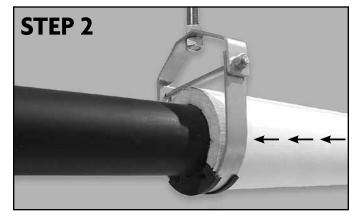
Slide the notched insulation section over saddle.
