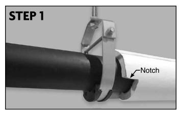
Cope or notch insulation to fit around saddle. The notch should be deep enough to extend  $\frac{1}{8}$  to  $\frac{1}{4}$  beyond the saddle.
