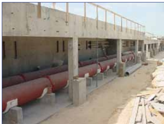
30" 7707L couplings on a chill water system
