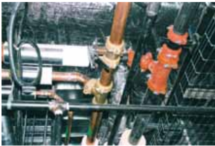
A SJ-C300 butterfly valve installed in a hot water system
