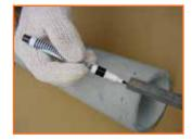
Marking Use a marker and measuring tape to place marks on each pipe end, 1" from each end.
