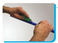
I. Cut and fold back plastic cover to reveal the copper tube
