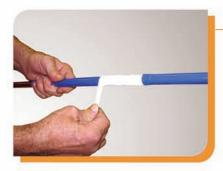
3. When the joint is complete and cool, replace the plastic coat and wrap the joint to give continuity of protection
