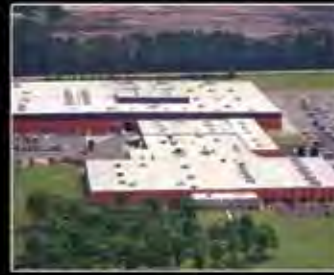
CONWAY, SC Steel Foundry and Manufacturing Plant
