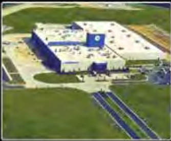
PAGELAND, SC Bronze Foundry and Manufacturing Plant
