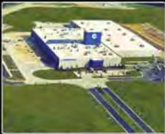
PAGELAND, SC Bronze Foundry and Manufacturing Plant
