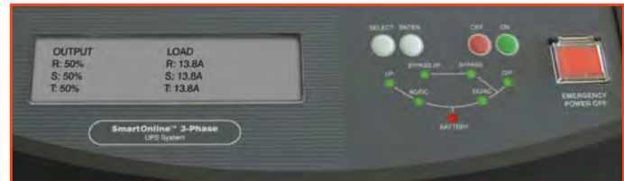
The LCD/LED control panel indicates more than 45 separate faults, warnings and operational conditions.
