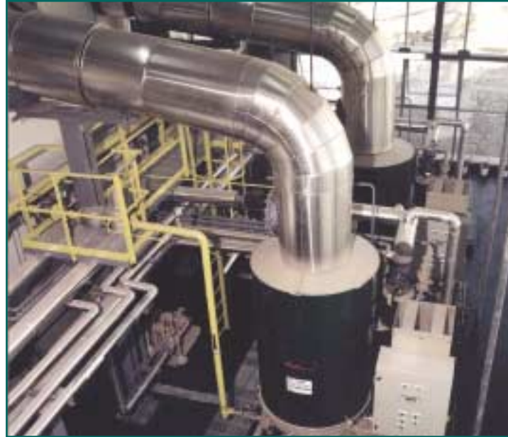
Two 300 BHP steam generators in a Romanian soap plant.
