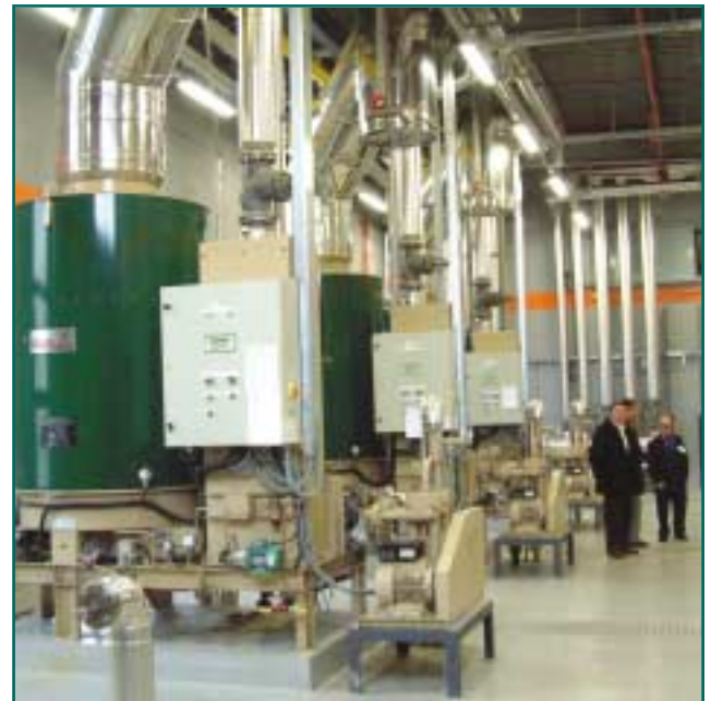
Three 350 BHP steam generators in a Spanish pharmaceutical plant.
