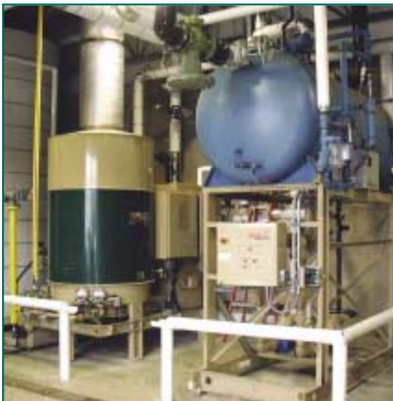
A 250 BHP steam generator in a U.S. food manufacturing plant.
