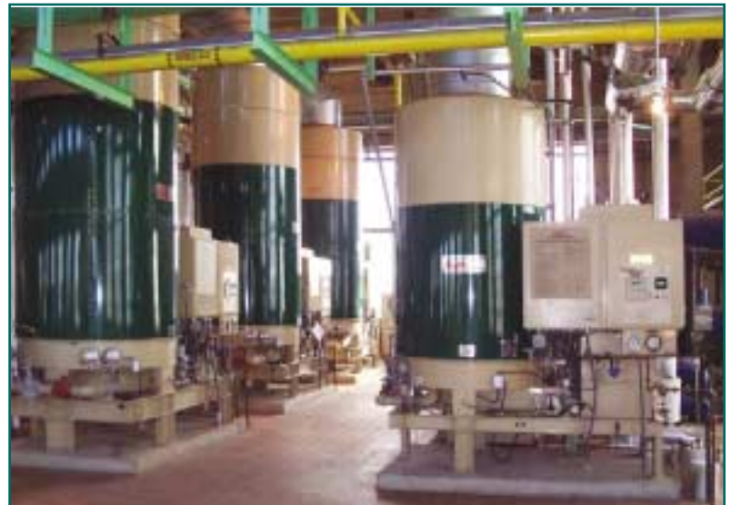
Three 600 BHP and one 300 BHP steam generators in a midwestern utility plant.
