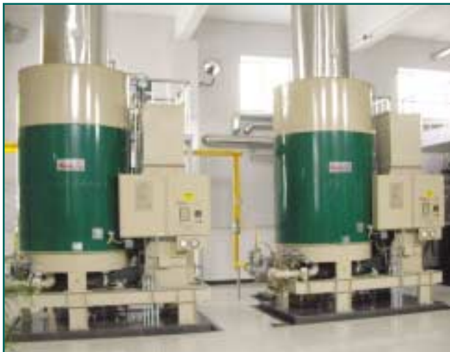
Beijing CCTV Installation.
