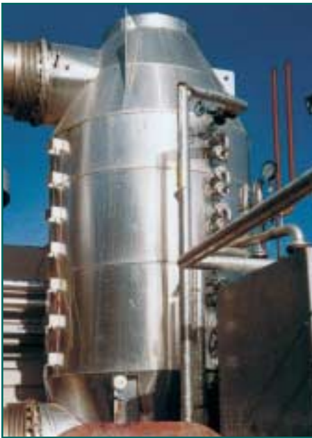
Exhaust Gas Boiler
