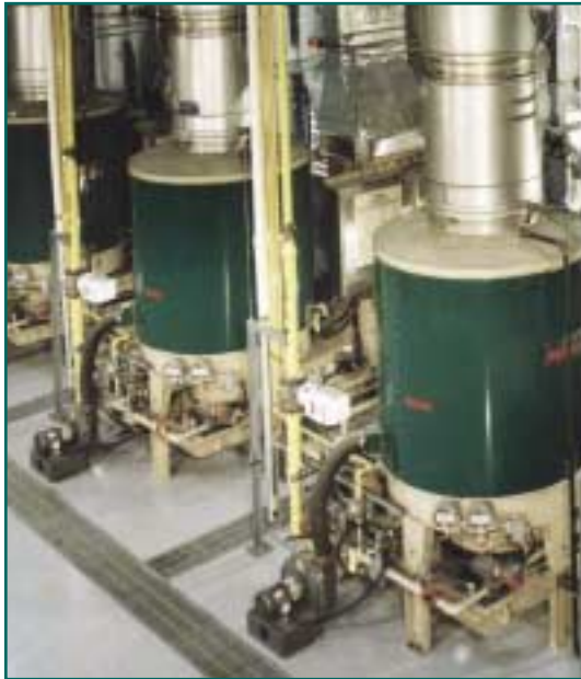
Three 250 BHP, 450 psig, steam generators in a steel vacuum de-gassing application.
