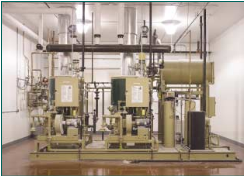
Two 100 BHP steam generators mounted on a single skid with the feedwater components operating in a U.S. candy manufacturing plant.
