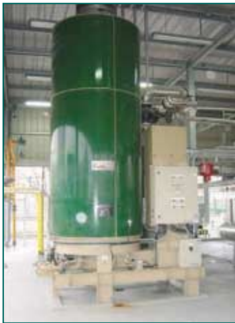
A 600 BHP Steam Generator in a U.S. Cosmetics Plant.
