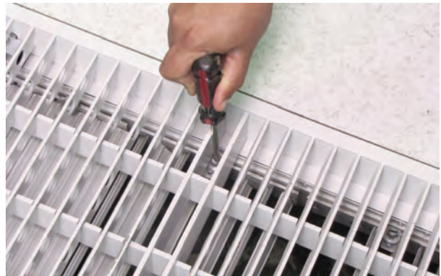
Adjust airflow without removing the DirectAire panel
