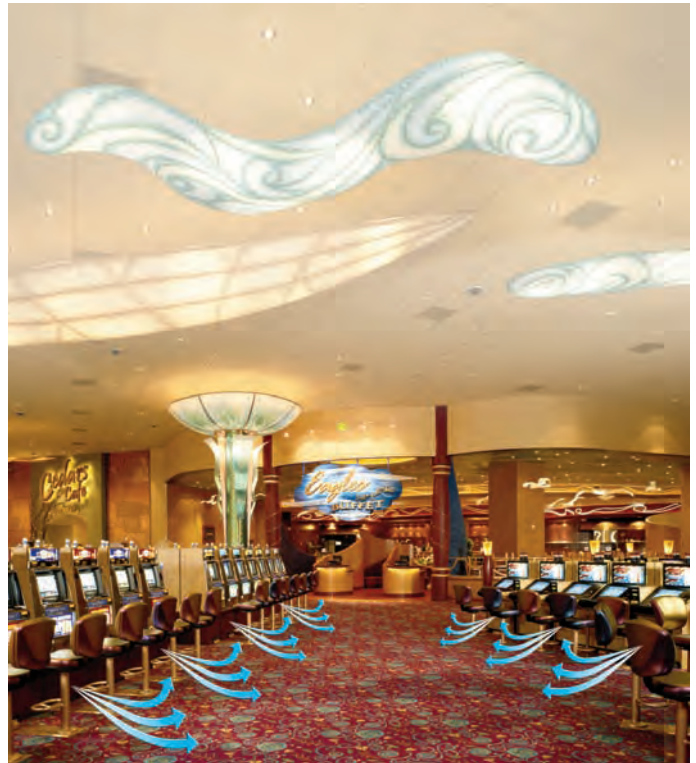
Underfloor Air Distribution with Air»Connect
