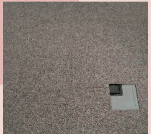
Step 6: Cut carpet tiles do not fit at new location, need new carpet tiles...
