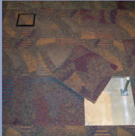
Step 2: Remove solid access floor panel....
