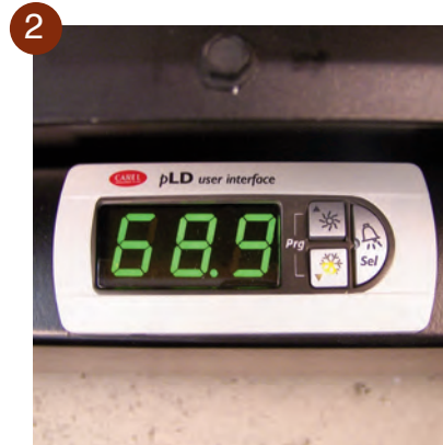
Temp Display and Setpoint Interface for SmartAire M & S
