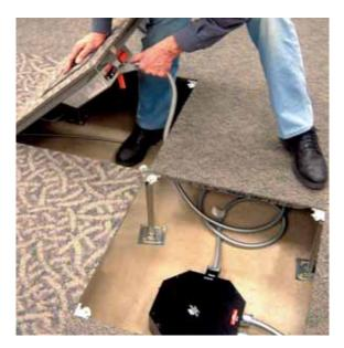
**Complete flexibility and reconfiguration capability** An access floor with modular 'plug & play' power wiring, and cabling components provides complete flexibility. As your business needs change so too can your service distribution system – quickly, easily and cost-effectively!
