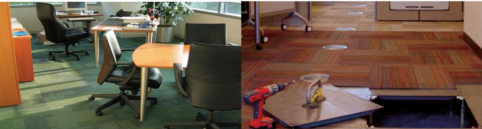
“ The full underfloor HVAC system uses fresh filtered air, which is distributed under the office floor. This allows occupants to control the air temperature of their workspace. ”
