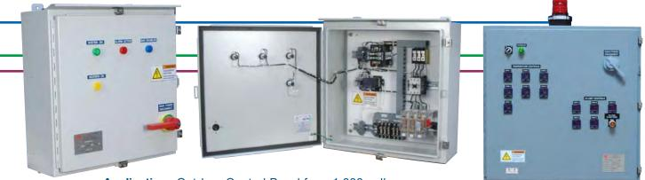
**Application:** Outdoor Control Panel for a 1,000 gallon water holding tank with internal temperature control, NEMA 4 construction and enclosure heater
