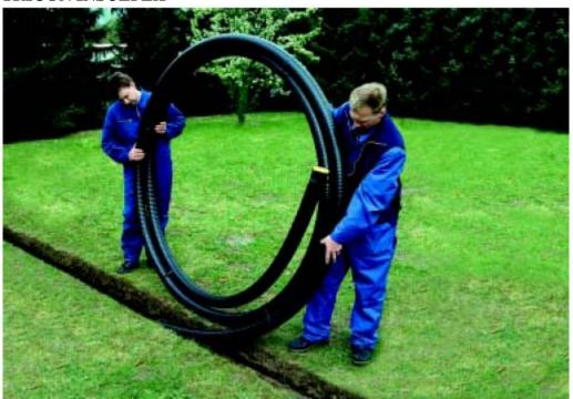
The transfer of hot or chilled water through buried pipelines requires a special piping system. TRICON INSULPEX is a preinsulated piping system that is not only flexible, but also has the ability to withstand harsh conditions.
