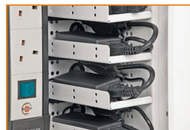
Power pack shelves located in the rear compartment provide excellent cable management
