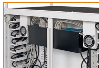
19" rack for mounting 2 network switches are provided for facilitating data transfer activities (Switched not included)
