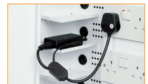
Power pack shelves and Y-leads provided for tidy storage and ease of use
