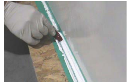
Figure 23: Horizontal finish with rounded corner
