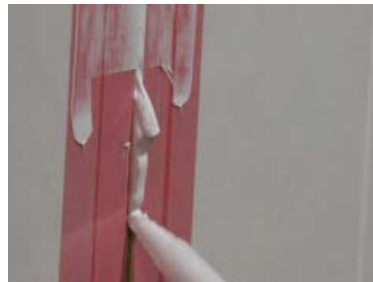
Figure 19: Bump adhesive in to previous section
