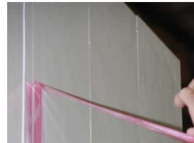
Figure 20: Removing Painter's tape
