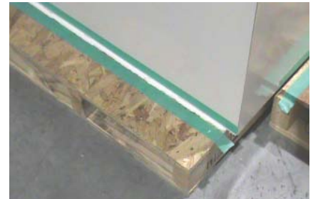
Figure 22: Horizontal seam filled completely with sealant
