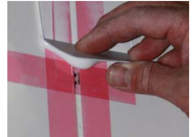
Figure 17: Applying the painter tape horizontal in 3' sections
