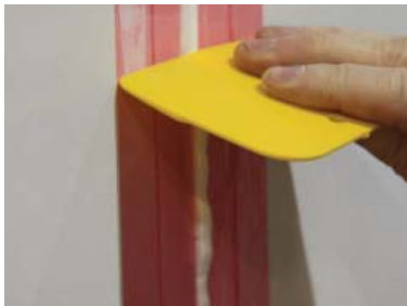
Figure 18: Removing excess sealant
