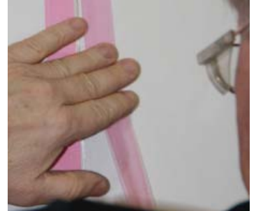
Figure 16: Applying the painter tape
