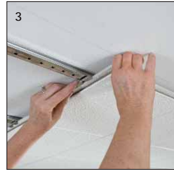
Step 3 – Position tiles or planks; slide and secure clip
