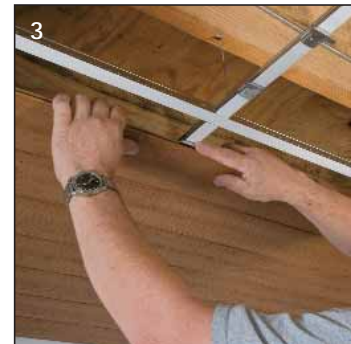
Step 3 – Position planks; slide and secure clips
