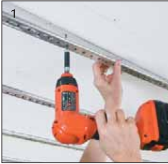
Step 1 – Attach tracks
