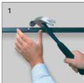
Step 1 – Install wall molding
