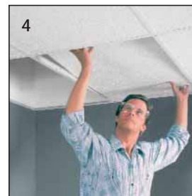
Step 4 – Install ceiling panels
