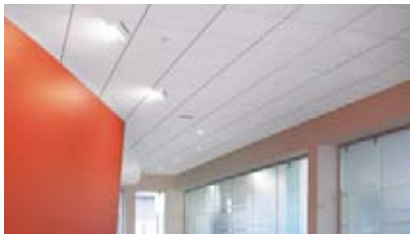
Flat, level ceiling with standard acoustical suspension
