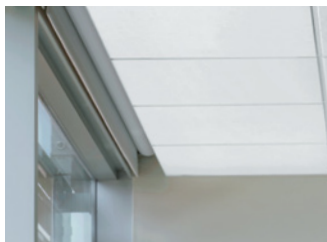
A Perimeter Pockets for a clean, seamless transition
