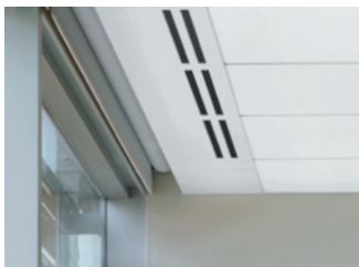
C For air distribution next to windows and walls, use slotted diffuser face plates
