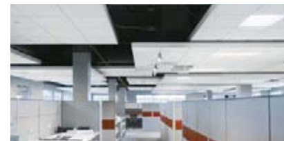
Flexible, safe low voltage power supply housed in ceiling clouds
