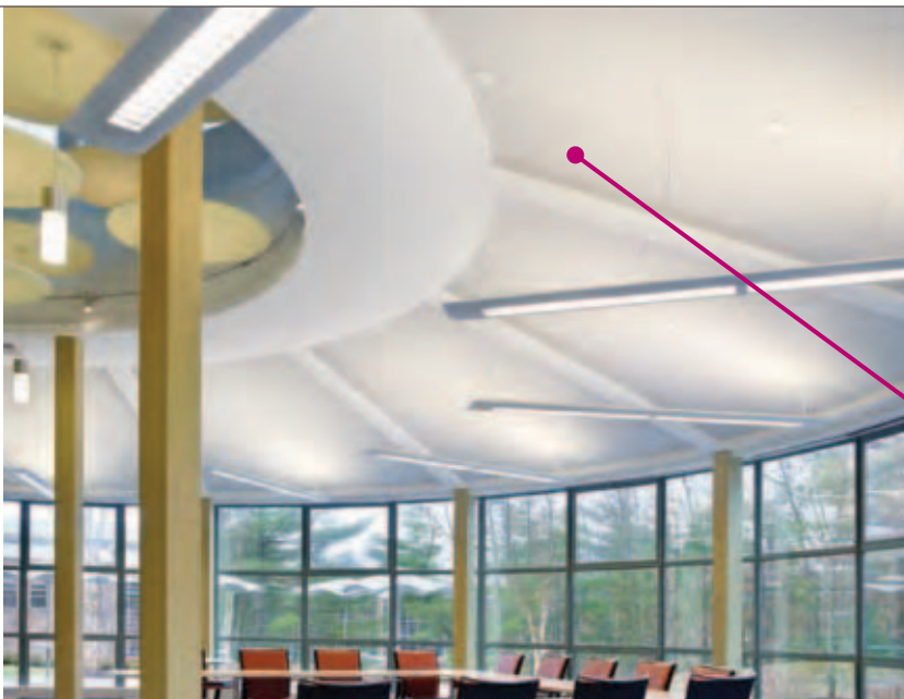
MetalWorks Radial RH200 Custom Ceiling System with Rd 1522 perforation in Silver Grey
