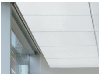
B For smooth changes in ceiling elevations, use Perimeter Pockets with extensions
