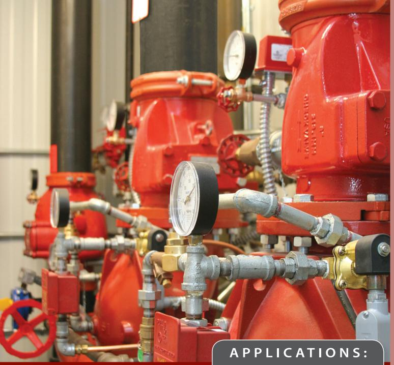
**General Purpose Valves** are for use in fire protection service applications where it is necessary to prevent reverse flow, or where system shut-off or sectional control is desired for closing a fire protection system after operation, or to facilitate testing.
