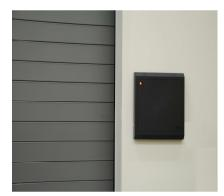
**Features** These readers contain (a) a 3-color LED to indicate successful card read and access-granted, (b) a 4 kilohertz beeper for attention and alarm, and (c) a "hold" circuit to delay data transmission. Both LED and beeper are controlled by the reader itself. All three functions can be controlled externally by the host system.
