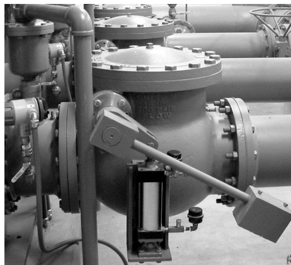
12" air-cushioned Swing Checks are shown at a recent Crispin installation. The air valves in the photo are also from Crispin.
