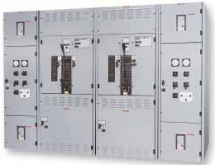
Fig. 5 Automatic transfer switchboard.
