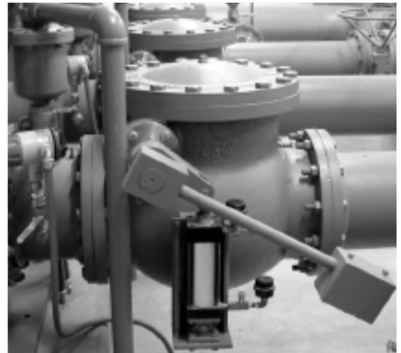
**12" air-cushioned Swing Checks are shown at a recent Crispin installation. The air valves in the photo are also from Crispin.**
