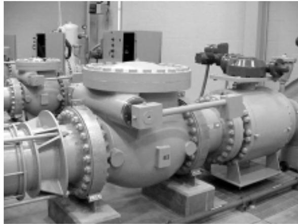
**Standard with Rubber Disc Seats and Stainless Steel Body Seats, Crispin Swing Checks are ideal for aggressive water and sewage applications.**
