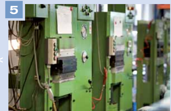
5 During the vulcanisation process the specific manufacturing parameters (for example: time, temperature, pressure, etc.) are monitored and recorded for future reference.
