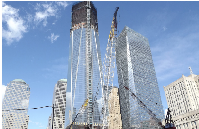
Freedom Tower installation
