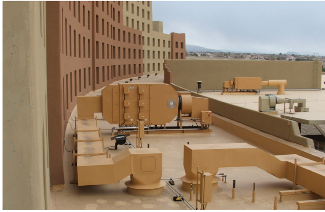
Sandia Resort & Casino installation
