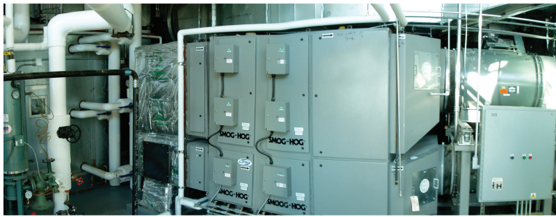
Hearst Tower installation
