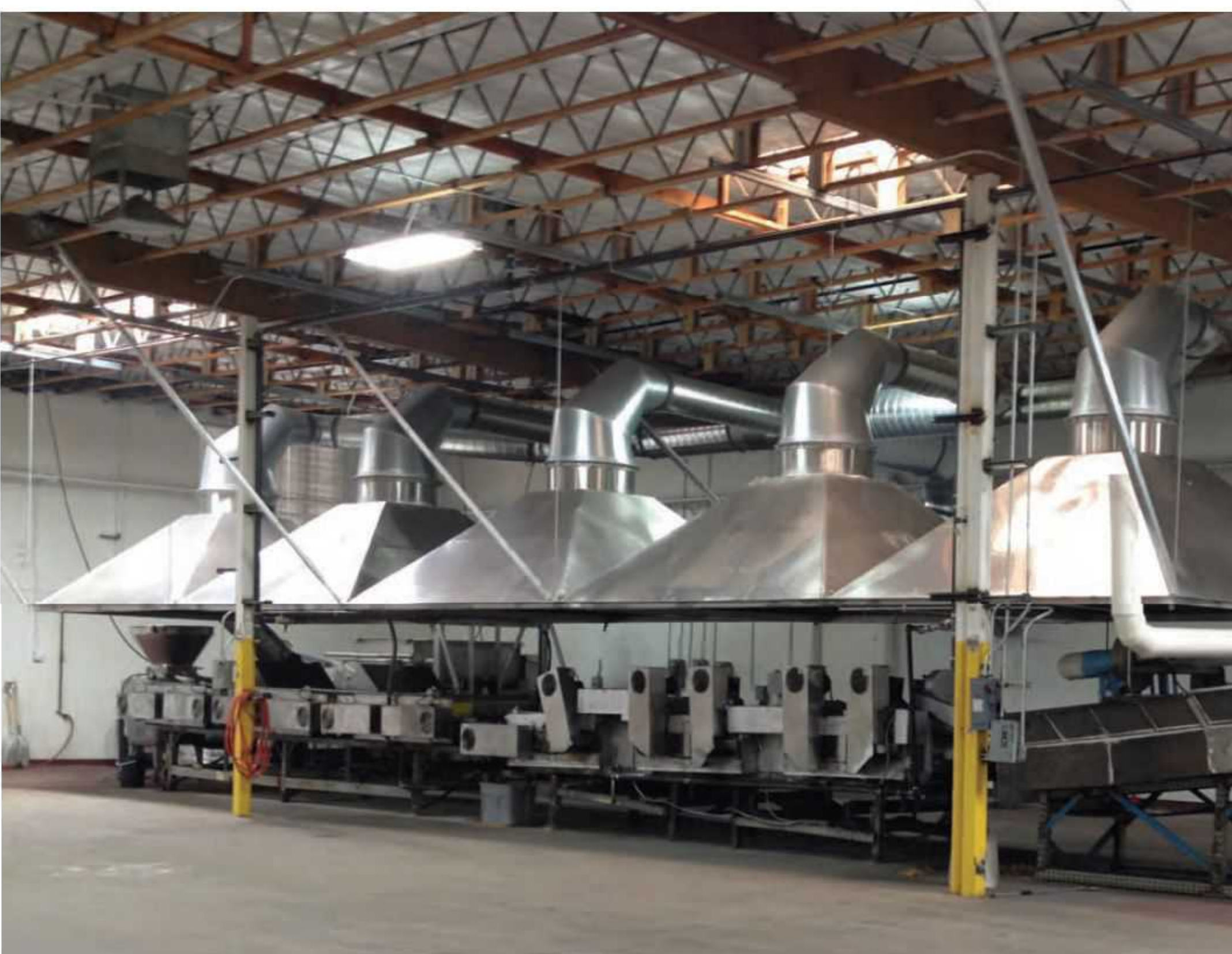
Five custom collection hoods built over the processing line to capture odor and smoke are ducted to the Smog-Hog unit outside.
