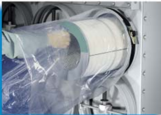
Model SFC bag-out collar filter change
