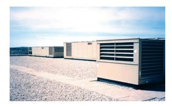
Rooftop units (RTUs) offer a simple and inexpensive solution to heating, ventilation and air conditioning (HVAC) for a wide variety of building types. Being the most commonly used HVAC system, RTUs are found everywhere from factories to schools, and commercial buildings to medical facilities.
