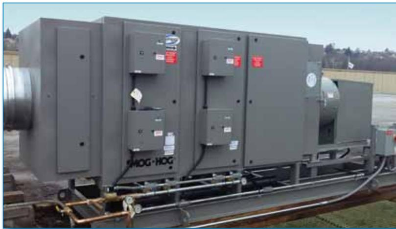
which also extend maintenance intervals. To control odor, UAS offers carbon or potassium permanganate filters. UAS systems are ETL listed and for an additional safety measure, the units can be equipped to work with Ansul fire suppression systems.
