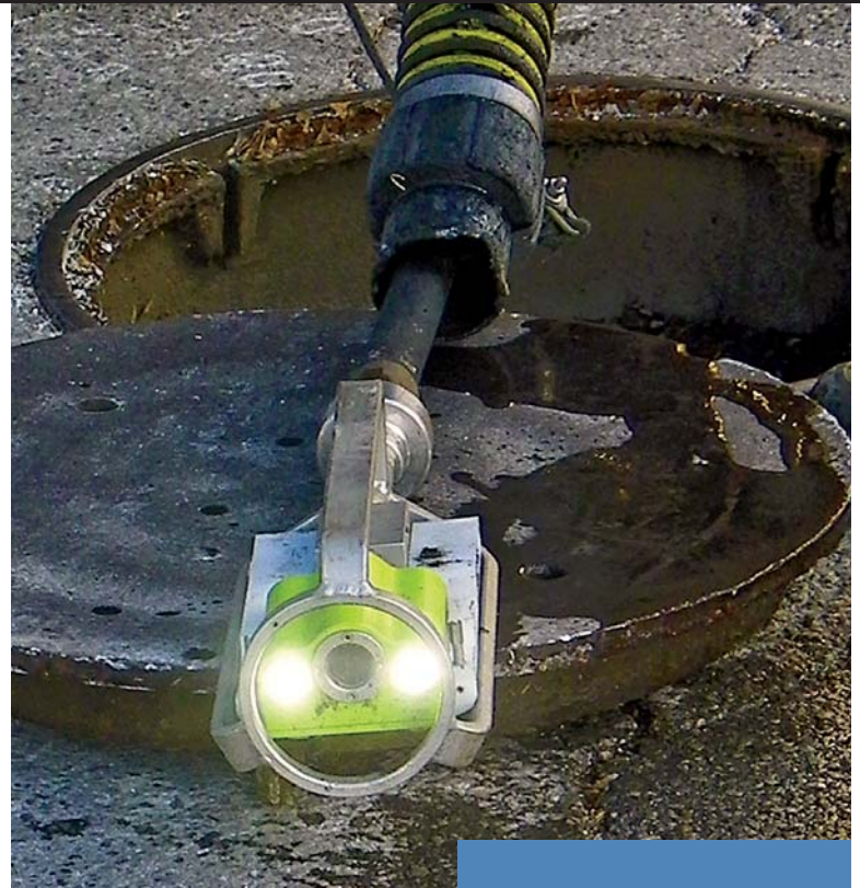
The JetScan is ready for deployment. The hose guard protects the jetter hose from chafing as it enters the potentially rough-edged sewer pipe. (Photography by Gil Longwell)
