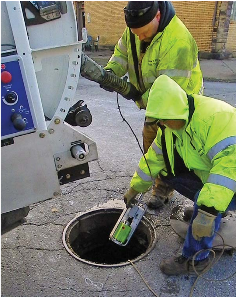
Beaver Falls Street Department crew members Bob Justisin (foreground) and Pat Burdine prepare to introduce the JetScan into the manhole.
