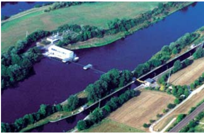
Ottendorf, Germany • Installer: Lingk & Sturzebecher.
