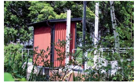
Typical pump house for the water hydraulic power pack.
