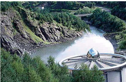
Naussac, France • Installer: Fluid Hydr'Eau.
