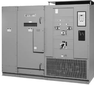
Indoor Unitized Power Center Bottom Cable Entry
