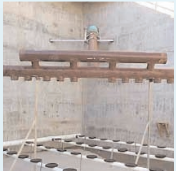
OMNIFLO® SBR with Fine Bubble Diffusers
