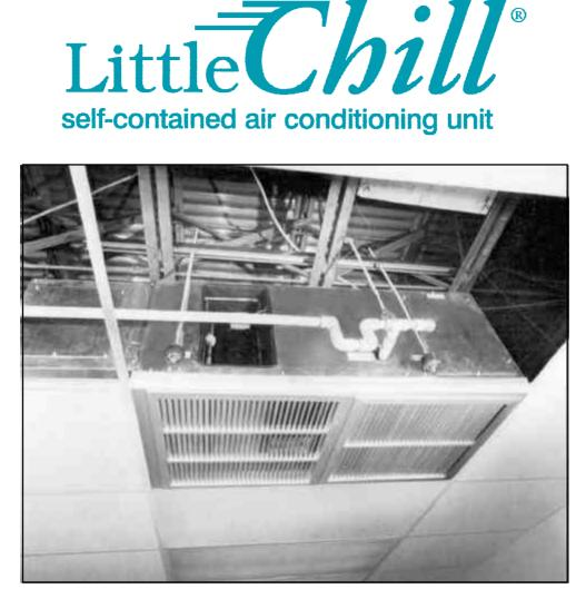
Little Chill Coolers from USA Coil & Air are the answer to your special cooling and dehumidification needs. For one thing, they fit right into a standard 2' x 4' suspended ceiling panel, with no floor space needed.
