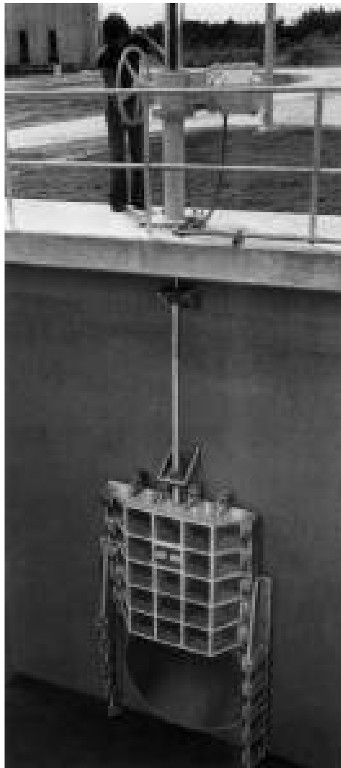
A typical sluice gate installation demonstrates how the various components of a sluice gate assembly are put together.
