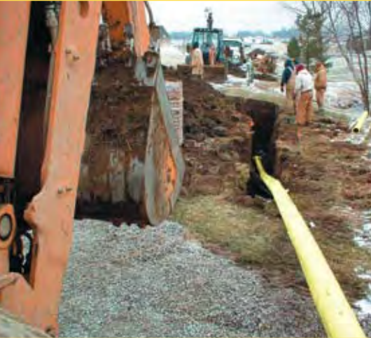
Yelomine IB trenchless installation
