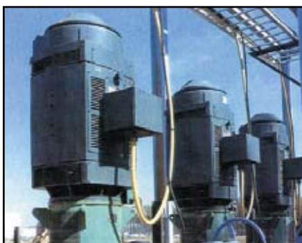
A clear water feed pump in a paper processing operation is driven by a Weather-Protected NEMA type 1 Duty Master Vertical Motor.
