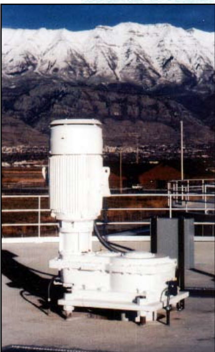
One of eight Reliance vertical P-Base motors in use at a wastewater treatment plant.
