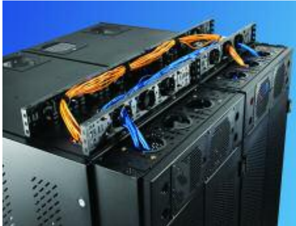
Strategically placed equipment, blocking panels and exhaust fans help to channel and remove heat from critical equipment bays.
