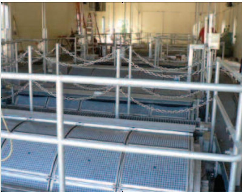
A B&G Booster Package provides pressurized water during the DrumFilter Backwash sequence.
