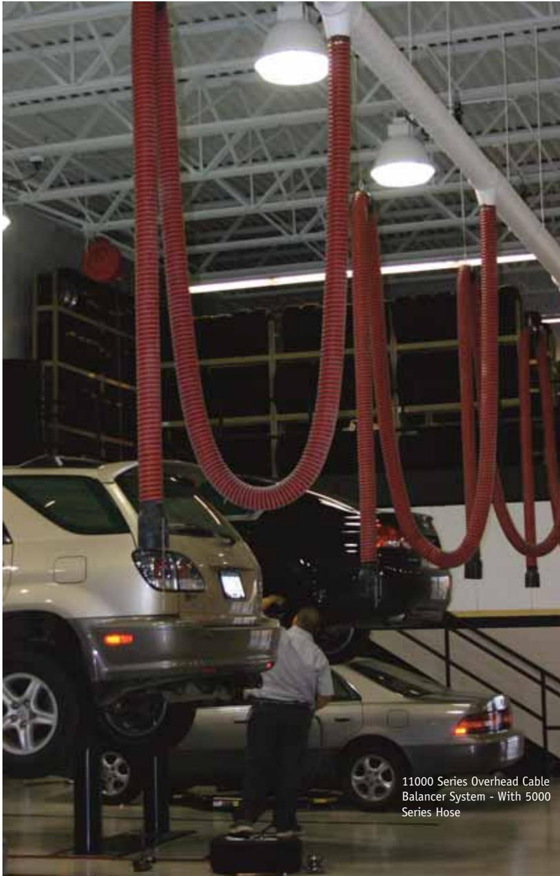
11000 Series Overhead Cable Balancer System - With 5000 Series Hose
